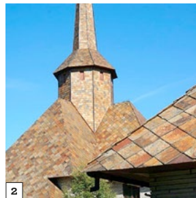
2. Dombås kirke. Rustfarget Ottaskifer. Dombås Church. Rust coloured Otta schist.
